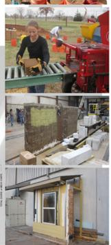
Series of images depict work days making Compressed Earth Blocks, structural test walls, and architectural mockup wall studies. Floor plan and wall section are referenced from student led construction documents (permit set).
